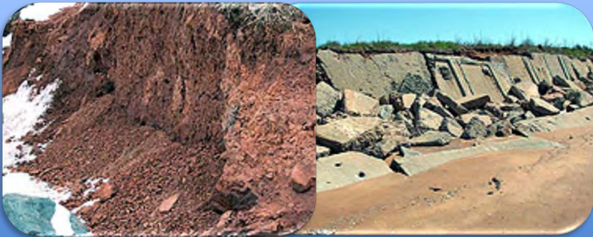
Figure 10 a and b: Property owners in Stratford, PEI, use cement blocks, wood beams, rocks and recycled build materials to build sea walls, in attempts to protect their lands from erosion.
