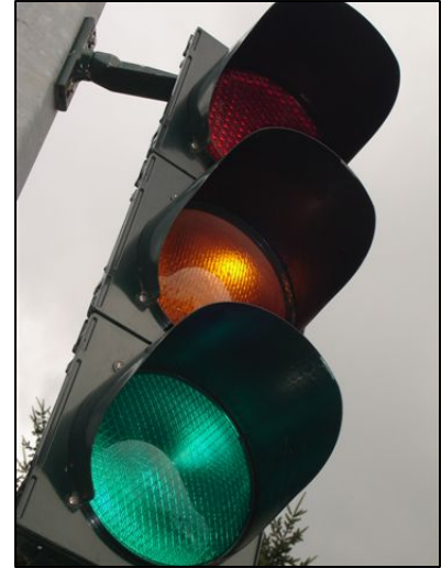
All signal lights have been replaced with energy efficient
