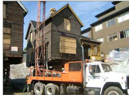
Figure 10. Installation of a geo-exchange system in New Westminster
