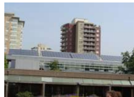
The North Vancouver public library has the most solar collectors of any building in B.C. Photo courtesy of the City of North Vancouver.
