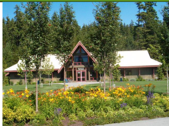
Top: Spruce Grove Field House. Left: The geo-exchange heat pump. Photos courtesy of the Resort Municipality of Whistler.
