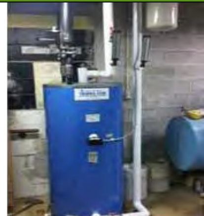
Water tank with d heat exchanger coil Photo courtesy of the City of Fredericton.
