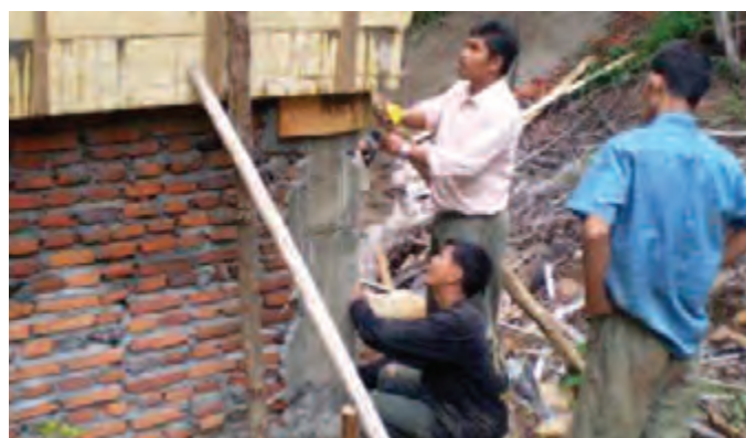
A CALGAP infrastructure specialist monitors a piping project in Aceh Jaya.
