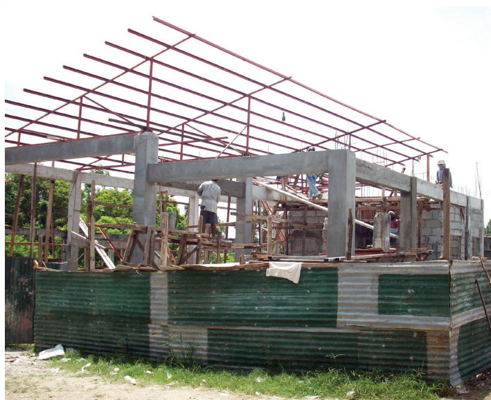
Construction of the new city fire department
